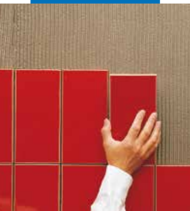
Fixing wall-tiles
