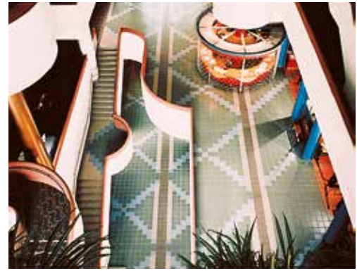
"Porcelain" quarry tiles laid with Kerabond + Isolastic - Civic Center - North York Ontario (Canada)
