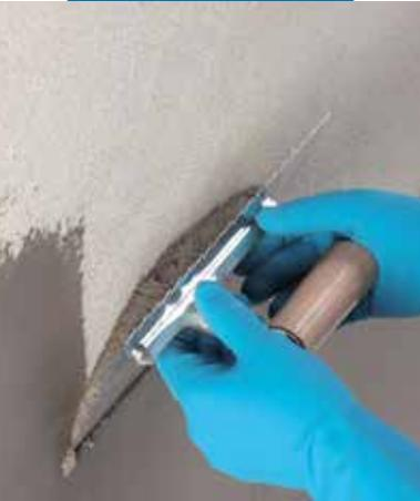
Spreading cement grey Fix & Grout Brick to a feather edge on the substrate
