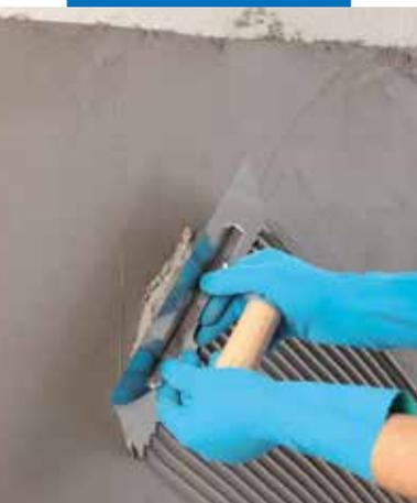
Spreading cement grey Fix & Grout Brick diagonally with a notched trowel
